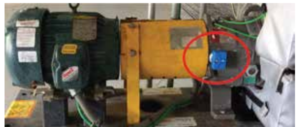
Figure 14: Chemical Process pump, side mounted to bearing frame
