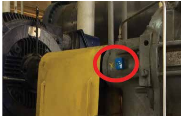
Figure 21: Vacuum Pump, side mounted to bearing housing
