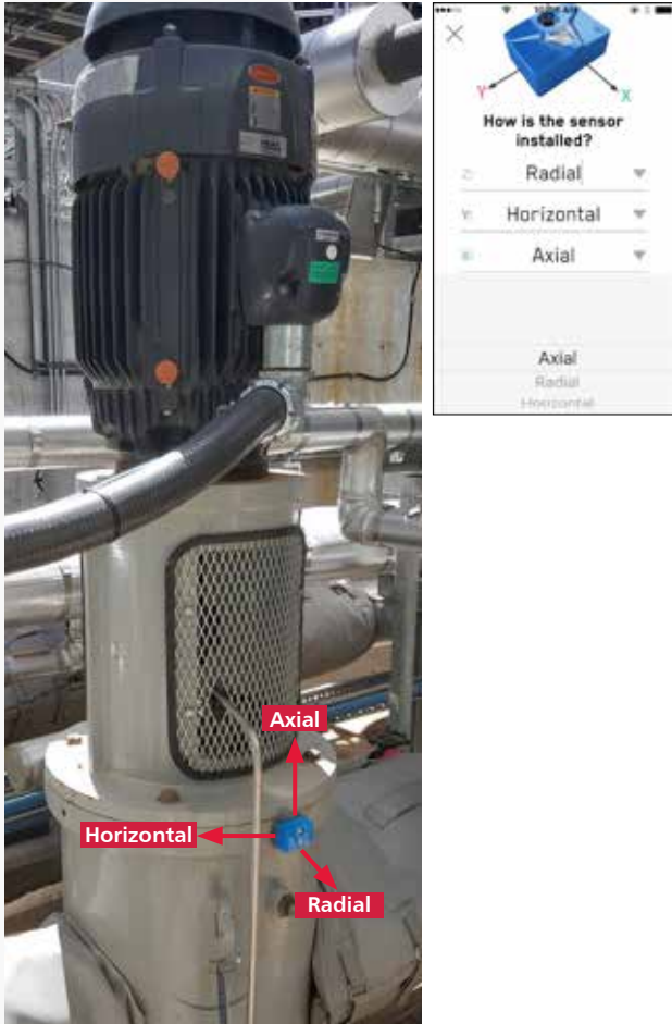
Figure 34: Standard orientation on a vertical pump
