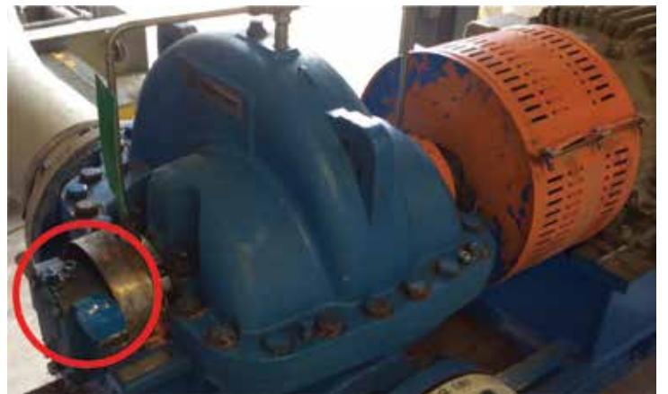
Figure 18: Double Suction, Horizontal Split case pump, mounted on thrust bearing housing
