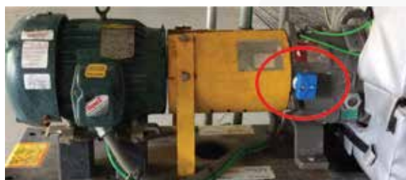
Figure 14: Chemical Process pump, side mounted to bearing frame
