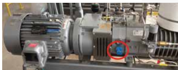
Figure 13: PD pump, side mounted to frame
