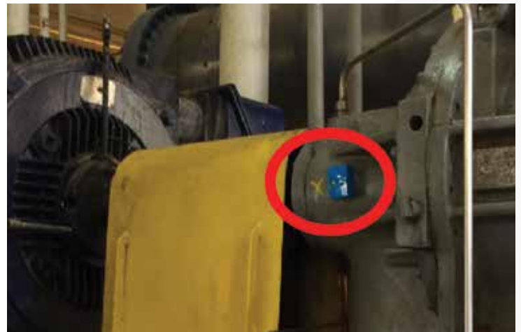
Figure 21: Vacuum Pump, side mounted to bearing housing
